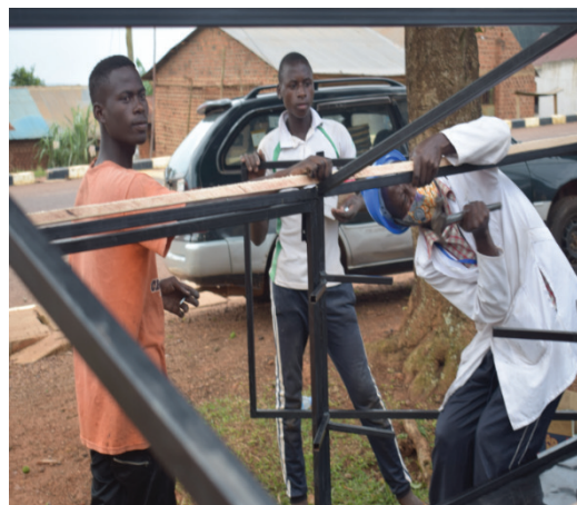
Figure 10 Joining small sized timber on the metallic frame of solar dryer
