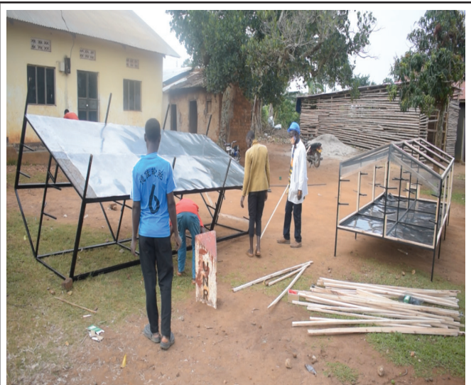
Figure 8 Inserting of a black iron sheet and painting of solar dryer
