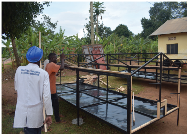
Figure 9 Adding timber on the solar dryer frame using nails and hammer
