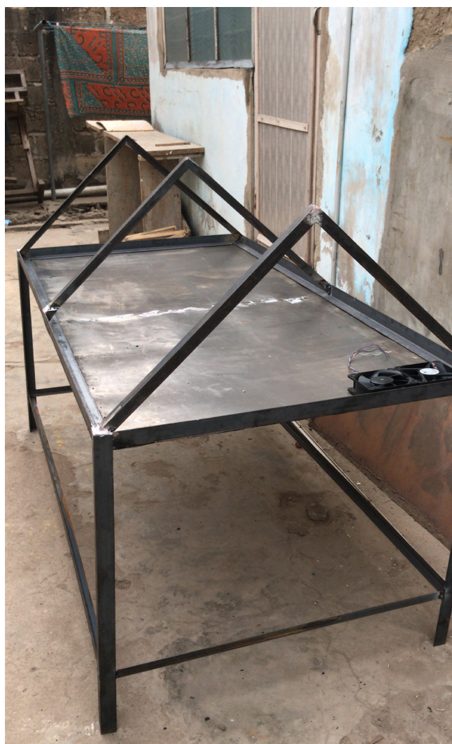
A frame of a mechanical solar dryer that is still under construction.
